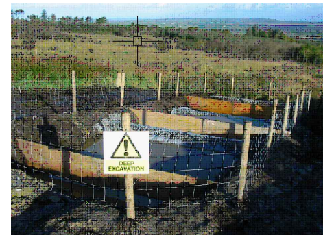
COMPLETED SETTLEMENT POND SYSTEM
